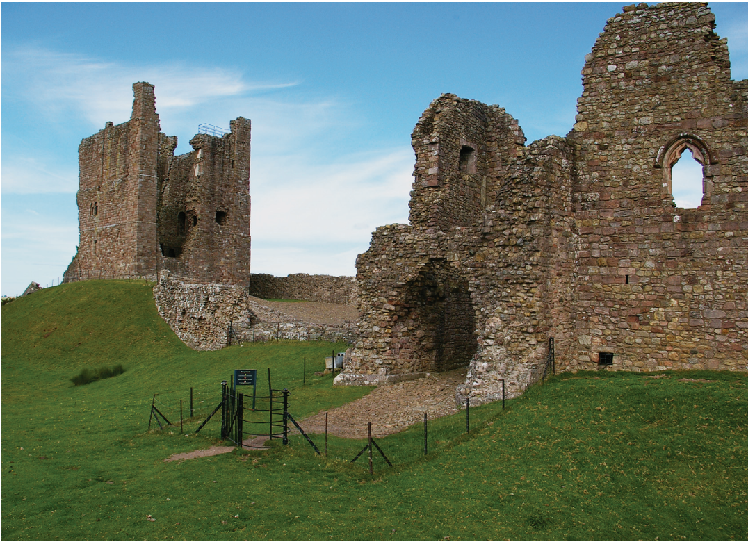
Plate III. Brough : Gatehouse and great tower from the SE.
